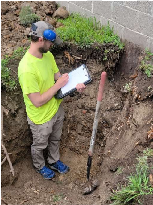
Justin from M&W sketches conditions 2' concrete wall above 2'-6" rubble "footing"
