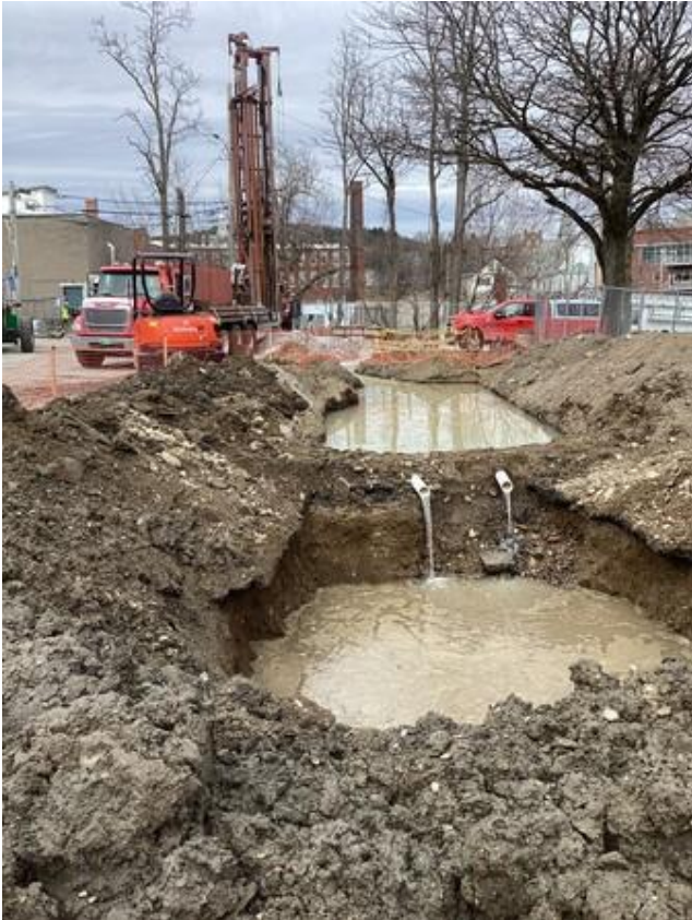
Geothermal well drilling, overflow containment basin
