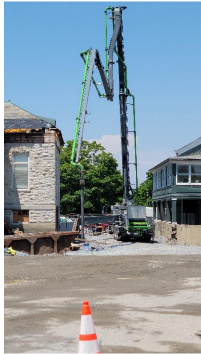
The Elevator Pit Triumvirate: ECI workers carefully tamp and measure depth of excavation, excavator operator removes material to waiting dump trucks, concrete pad and walls are formed and poured via pump.
