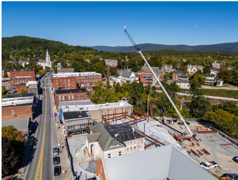
View of the crane setting the steel structure for the addition. Photo by Eric Killorin.
