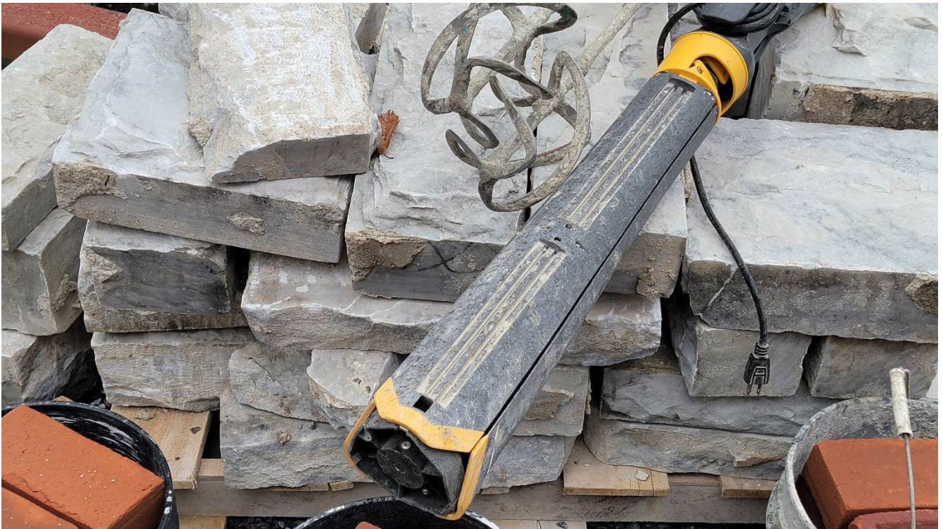
Tedesco Masonry has salvaged sufficient south wall original marble facing for re-use on north wall infills.
