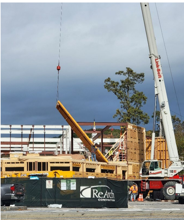
Second floor walls taking shape! Roof CLT next .
