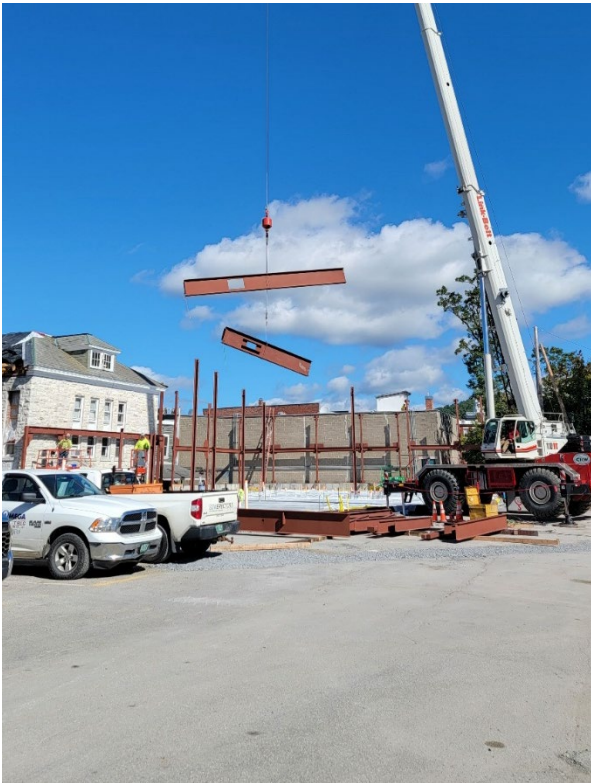
Steel installation! Beams “flying” to SSW Erectors.
