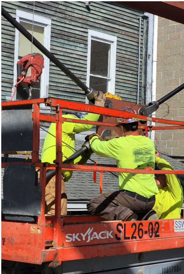
Electronic “yarning” of a massive cross-brace into place.
