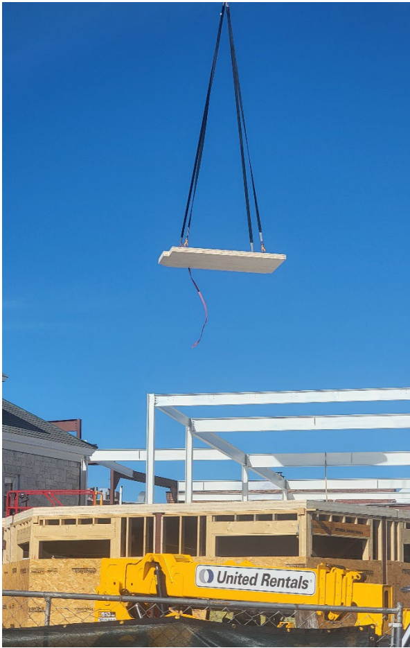
“Flying” the CLT panels– crane operator’s skills on exhibit.
