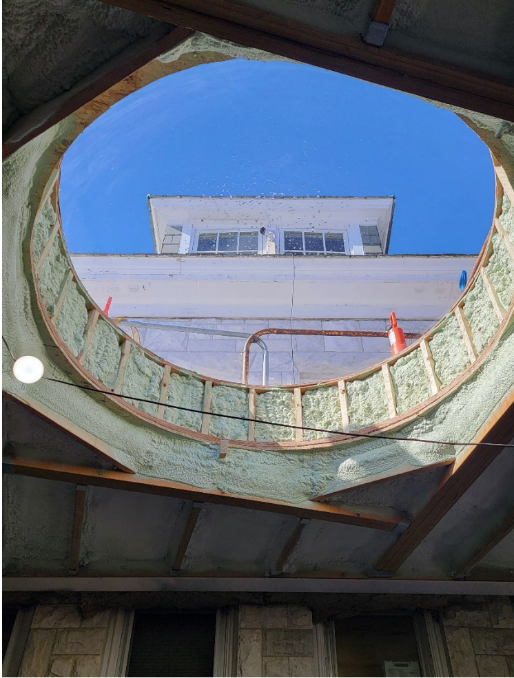
Atrium triple pane dome skylight in place. 1924 building east dormer perfectly framed above.
