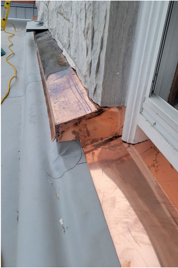
Copper flashing details at expansion joint between 1924 building and roof terrace. AC Hathorne team at work carefully creating and fitting pieces from flat stock.
