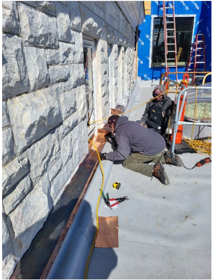
Copper flashing details at expansion joint between 1924 building and roof terrace. AC Hathorne team at work carefully creating and fitting pieces from flat stock.
