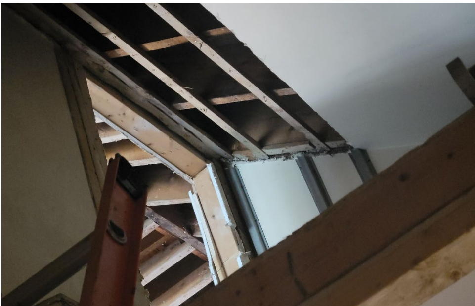
Atrium triple pane dome skylight in place. 1924 building east dormer perfectly framed above.
