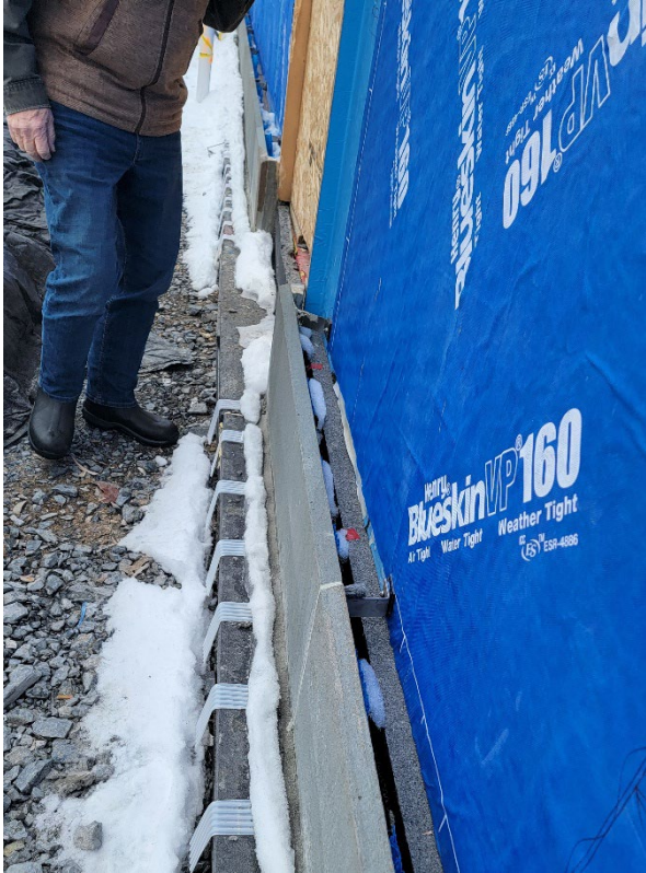
BLUESTONE damp course (base course) in place. TEST FIT! EDI crew hangs the first piece of terracotta. Perfectly level, plumb, and true! March 05, 2026.
