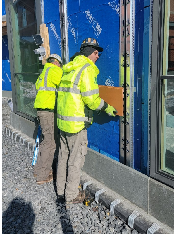
BLUESTONE damp course (base course) in place. TEST FIT! EDI crew hangs the first piece of terracotta. Perfectly level, plumb, and true! March 05, 2026.
